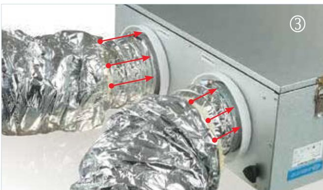
Tuck the inner insulation layer of the air ducts under the flanges of NM Isovent mounting kit.
